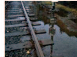
Track at end of replacement
