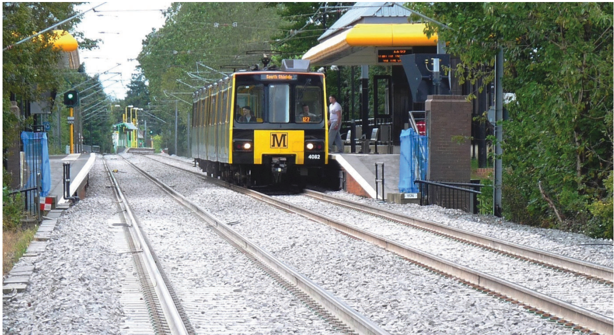
Refurbished Metrocar at the refurbished Meadowell Station on new track
