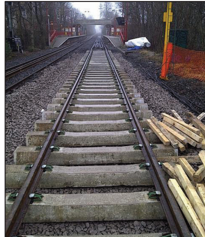
3) Plain line renewal at Hadrian Road, looking towards Wallsend. The image shows the new ballast and track (the light grey area on the left) compared to the old ballast, where the track has just been removed, on the right. Below – new track
