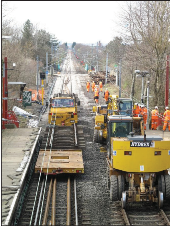
3) Plain line renewal at Hadrian Road, looking towards Wallsend. The image shows the new ballast and track (the light grey area on the left) compared to the old ballast, where the track has just been removed, on the right. Below – new track
