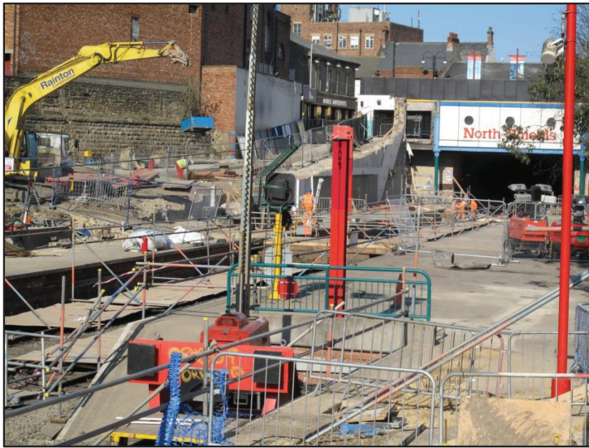
8) North Shields general view of demolition work
