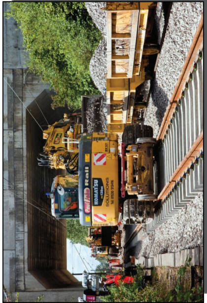
Track replacement between North Shields and Hadrian Road
