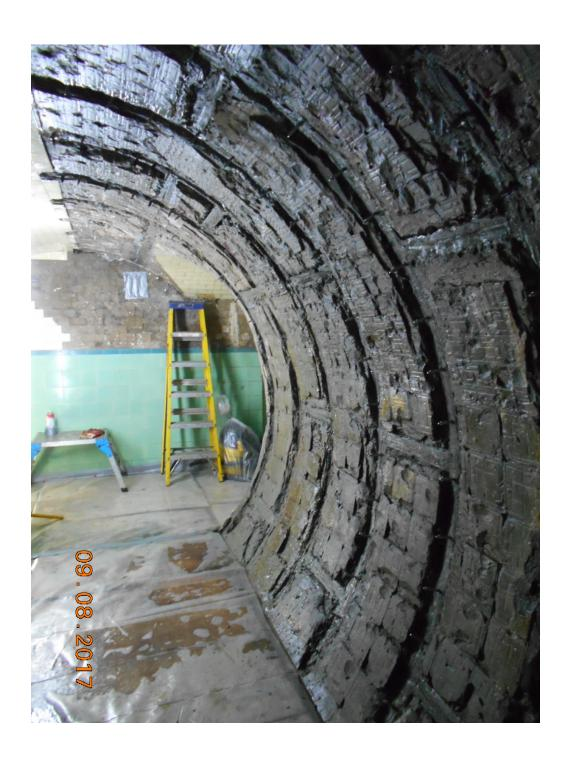
The existing tiling has been removed from the walls of the link corridor from the pedestrian tunnel to the vertical lift to allow resin injection works to be carried out to prevent water penetration into the tunnels. Once dry these walls will be retiled.
