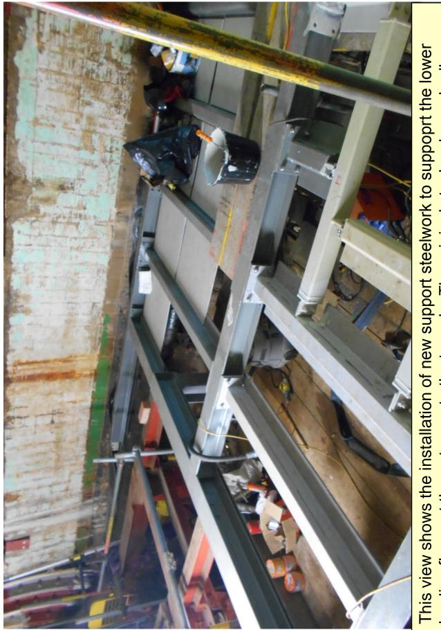
landing floors at the entrance to the tunnels. The original steelwork was badly corroded and had to be replaced.
