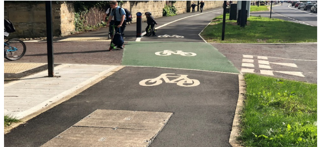
Tranche 1: Broadway to Brunton Lane Cycle Scheme in Newcastle
